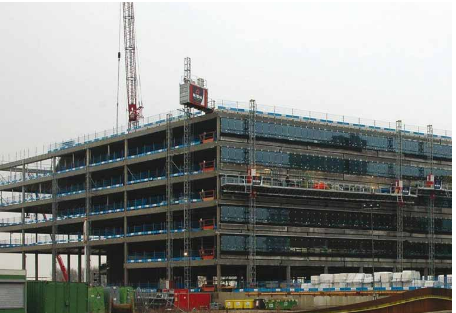
Ruwbouw is in volle gang
