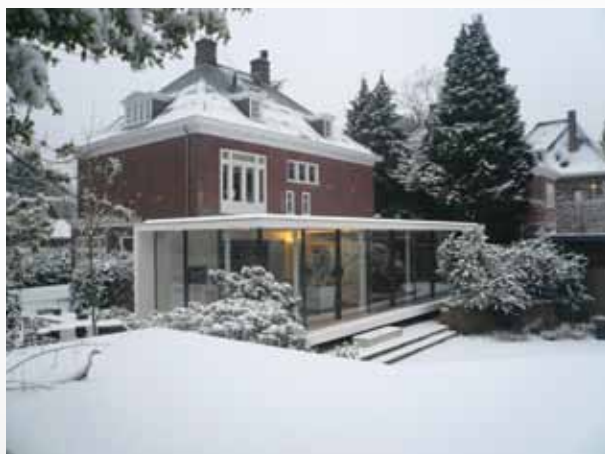
Villa in Hilversum Architect: Guller Guller Architecture Urbanism, Rotterdam
